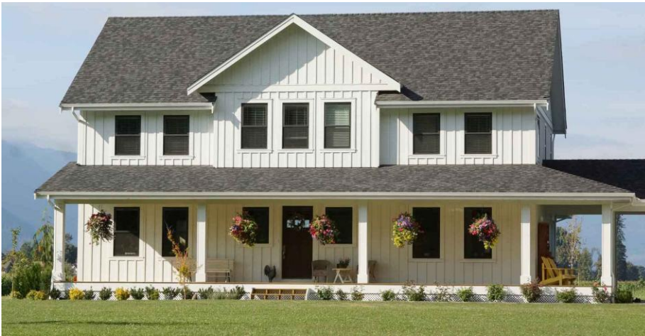
Board and Batten style steel panels
