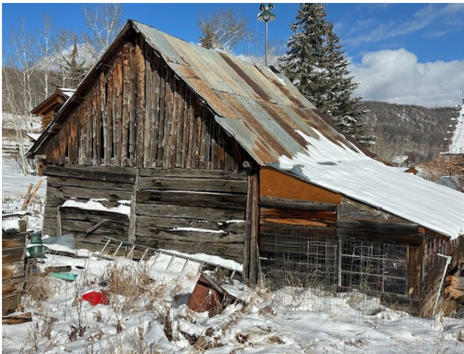
Figure 6. Rear view of shed showing loading shed addition, 2025.
