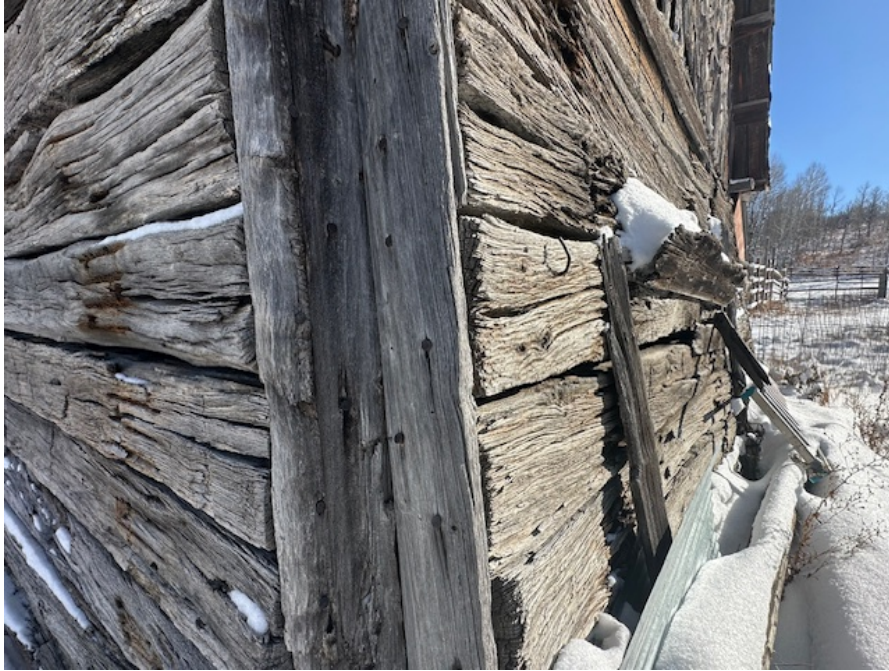
Figure 7. Shed corner showing railroad ties and hog trough corner, 2025.
