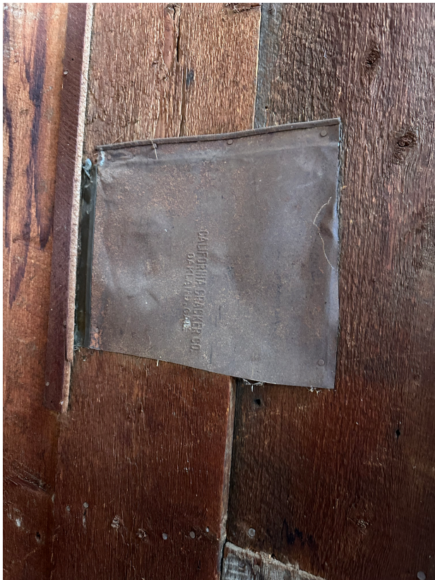
Figure 8. Detail of shed's interior vertical boards and metal patch, 2025
