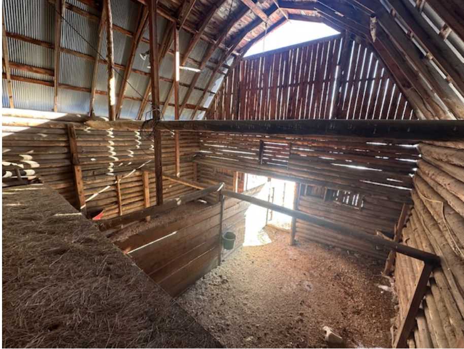
Figure 3. Barn interior from hayloft showing construction of roof and gable end, 2025.
