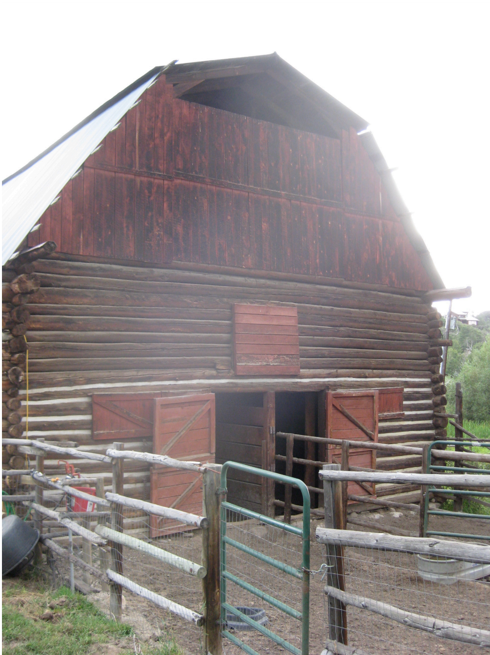
Figure 2: Rear entrance of barn showing portion of corral, 2011.
