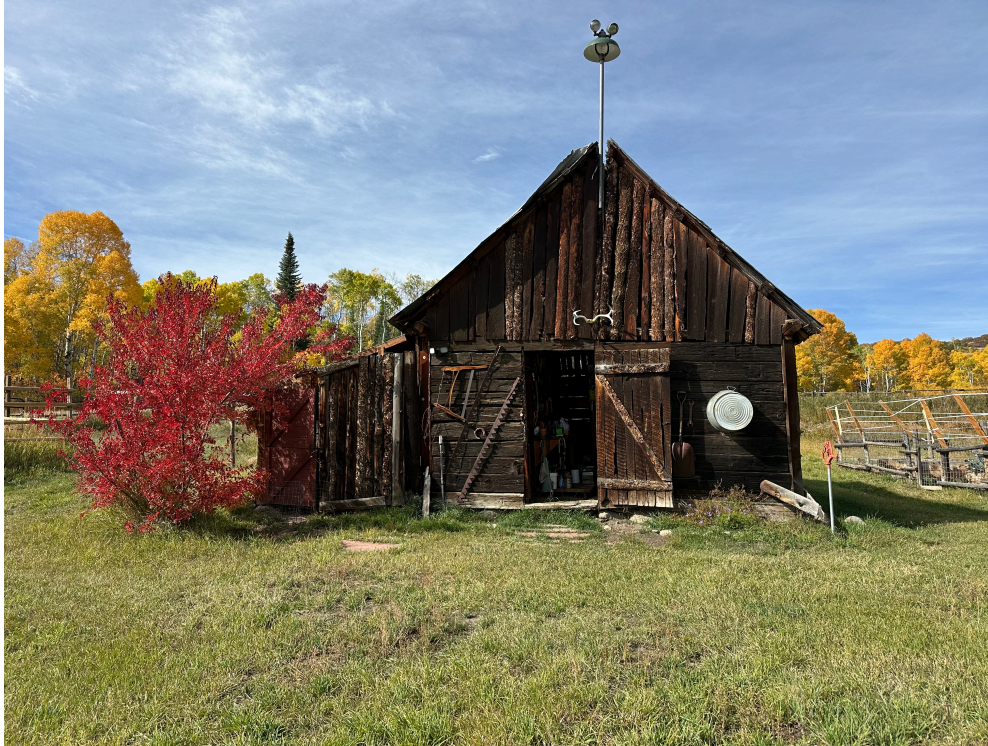
Figure 5: Front view of shed with vintage yard light attached to front gable, 2025.
