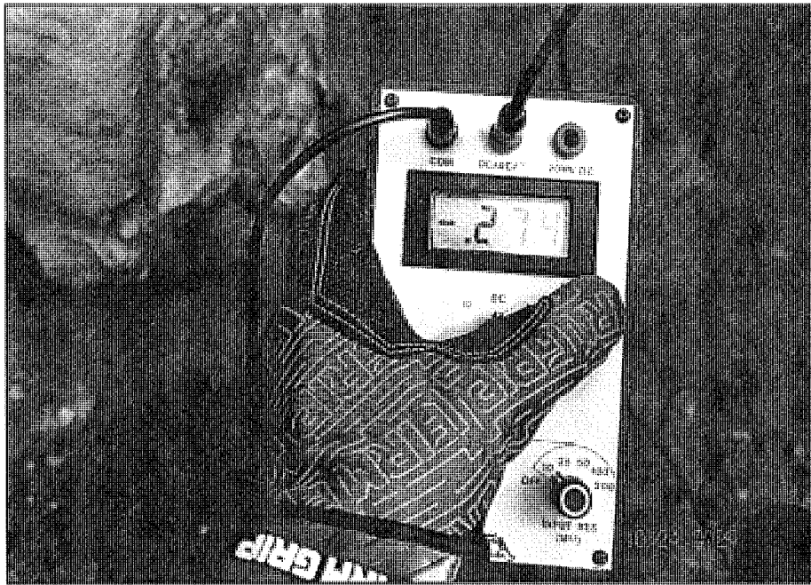
PHOTO NO.11: Photographic representative half-cell potential for corrosion reading.
