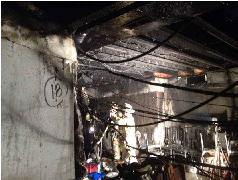
Figure 3: Crews in basement performing overhaul.
