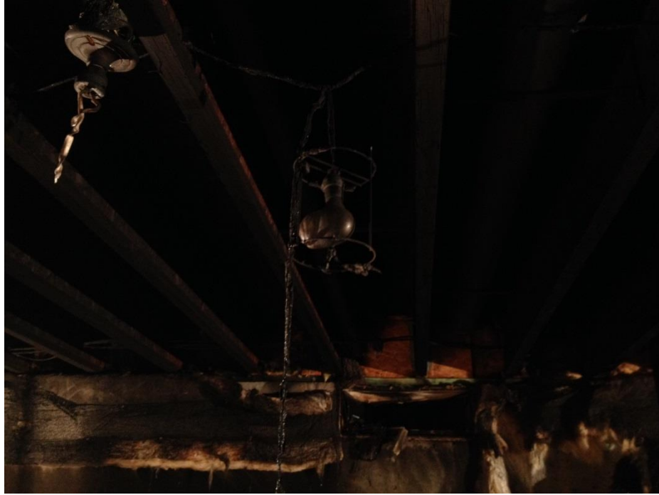
Figure 4: Light bulb distortion from fire development in basement.
