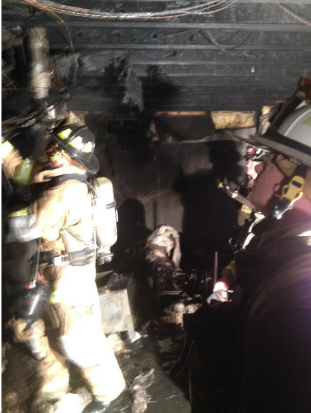
Figure 2: Crews pulling ceiling in basement.
