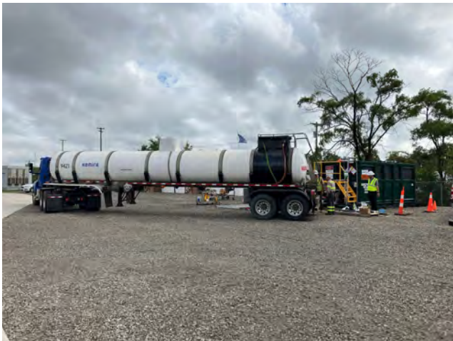
Ferric Chloride dosing will help alleviate adverse odors from the diverted flow.
