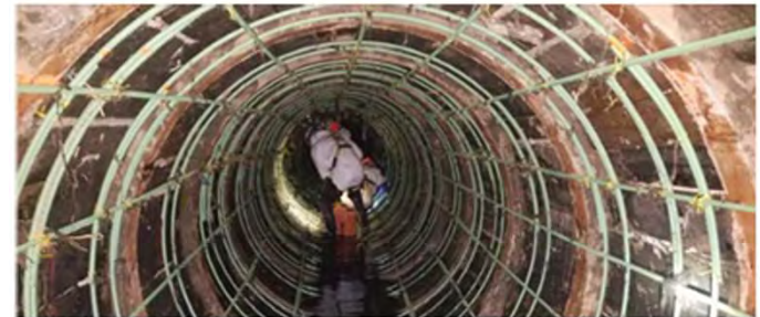
CON-149, Emergency Sewer Repair
