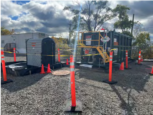
Ferric Chloride dosing will help alleviate adverse odors from the diverted flow.
