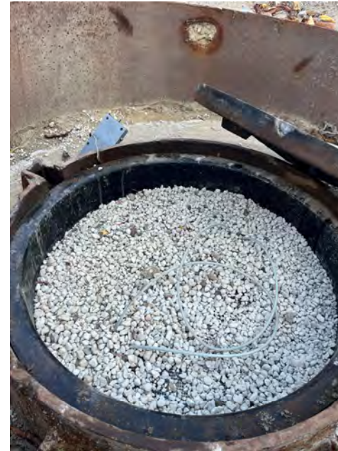
GLWA installed a manhole scrubber that provides passive, low-maintenance odor treatment.
