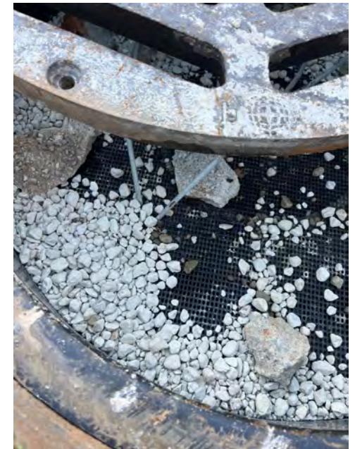
GLWA installed a manhole scrubber that provides passive, low-maintenance odor treatment.
