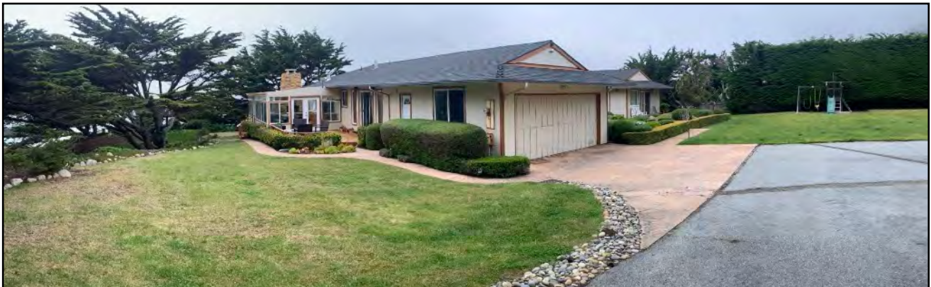
East and south side of existing residence.
