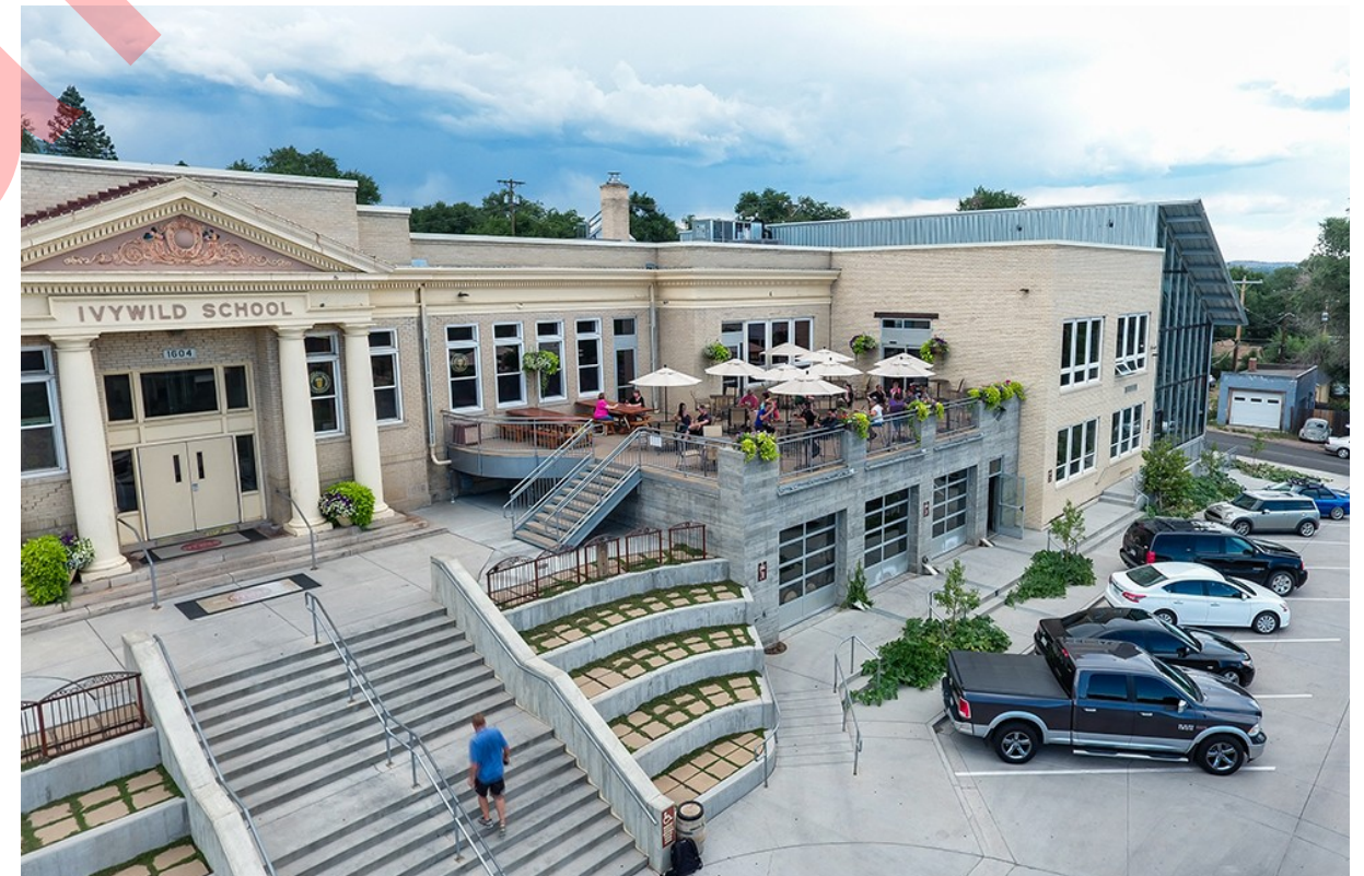
The Ivywild School is a successful adaptive reuse project that was redeveloped into a mixed-use facility with CDBG funding.
