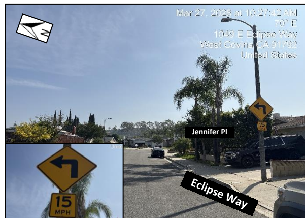
Curve Warning Sign & "15" MPH Advisory Speed along eastbound Eclipse Way, approaching Jennifer Place.
