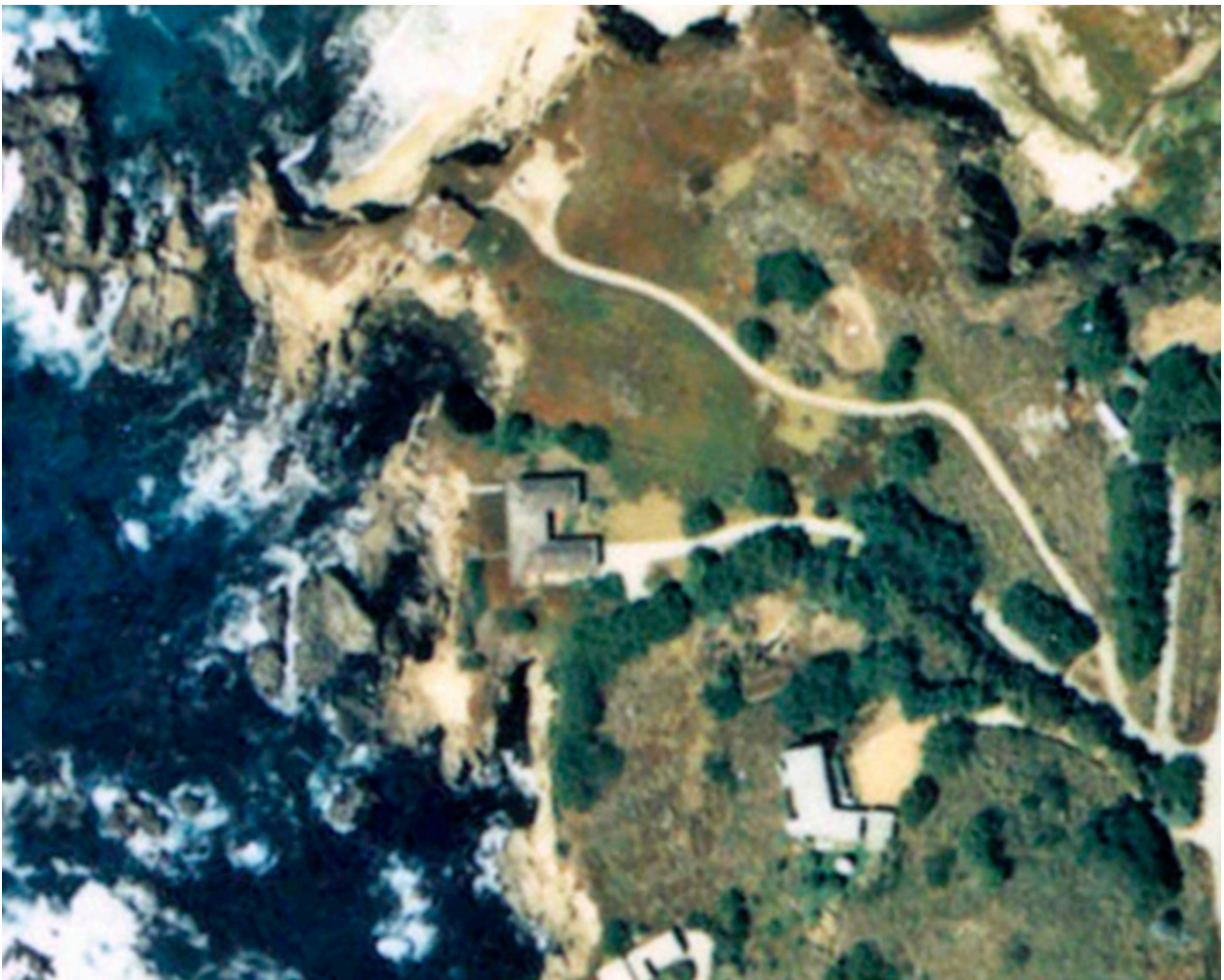
1986 Vertical Aerial Photograph of 35700 Highway 1
