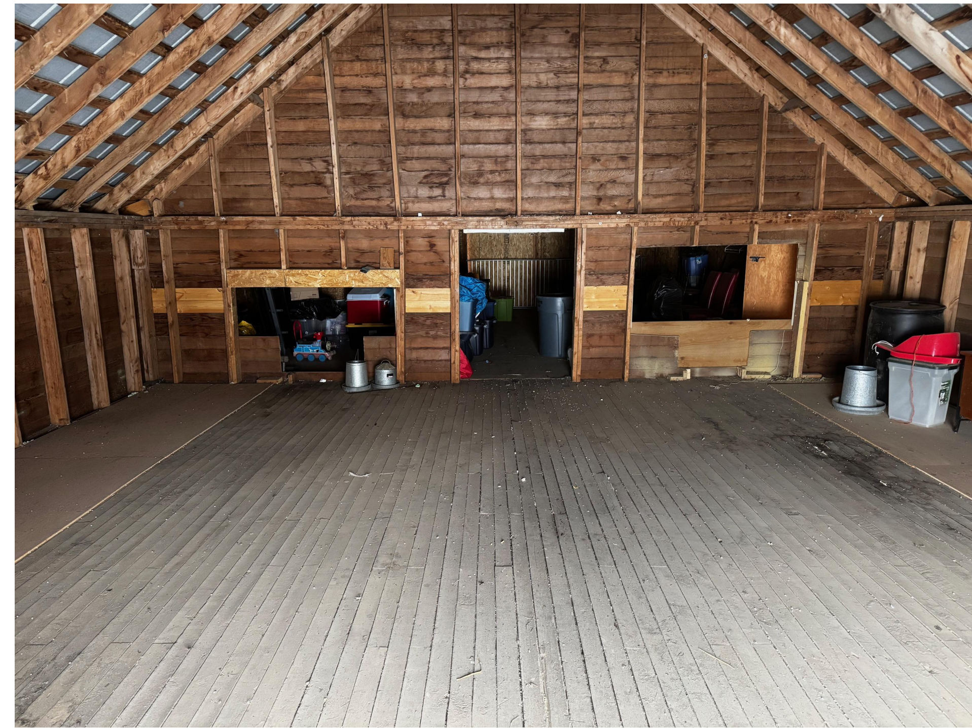
SOUTH BARN INTERIOR
