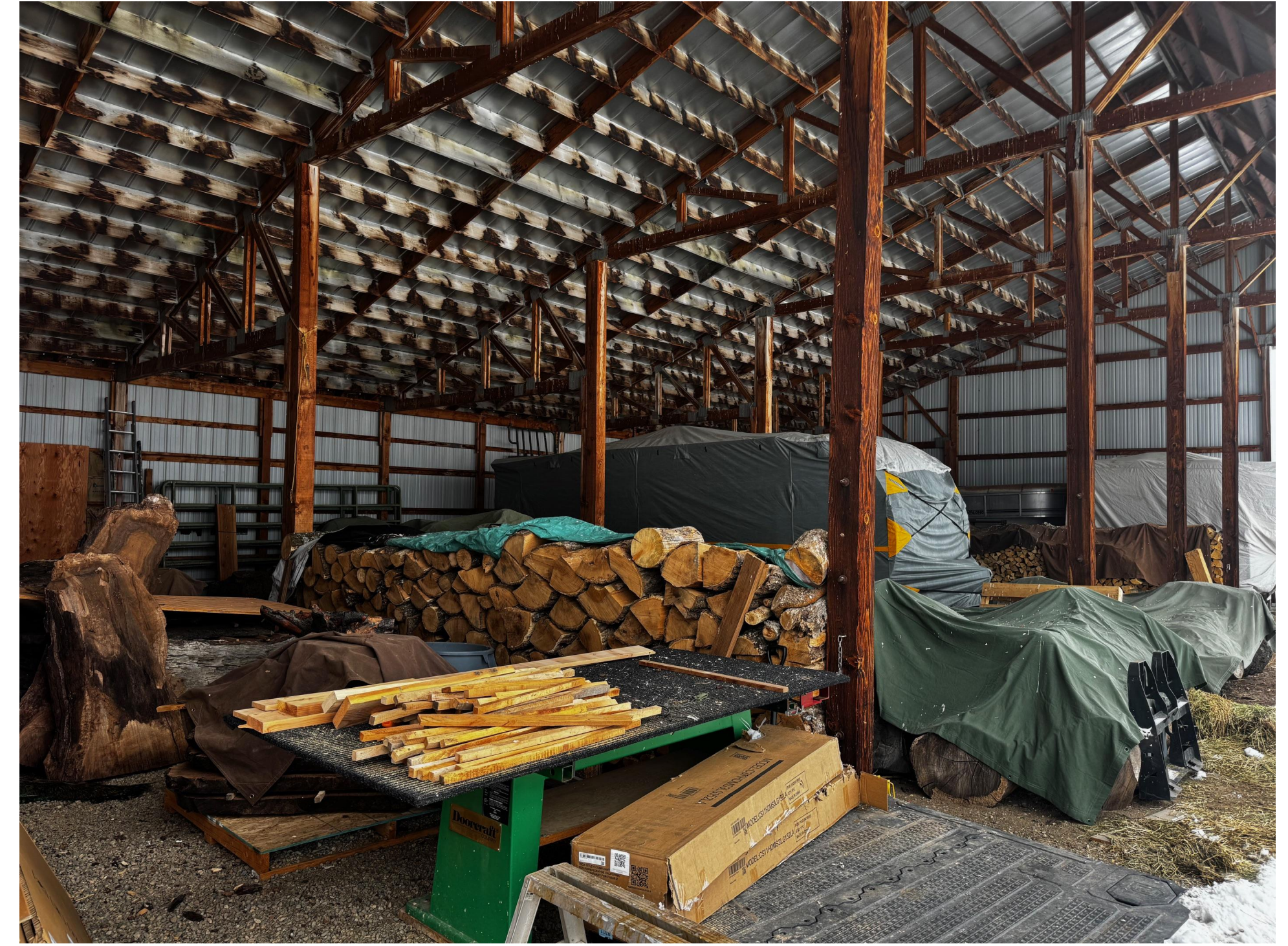
SOUTH BARN INTERIOR
