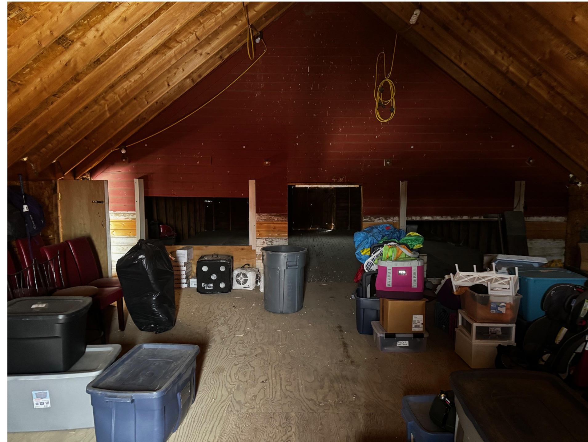
SOUTH BARN INTERIOR
