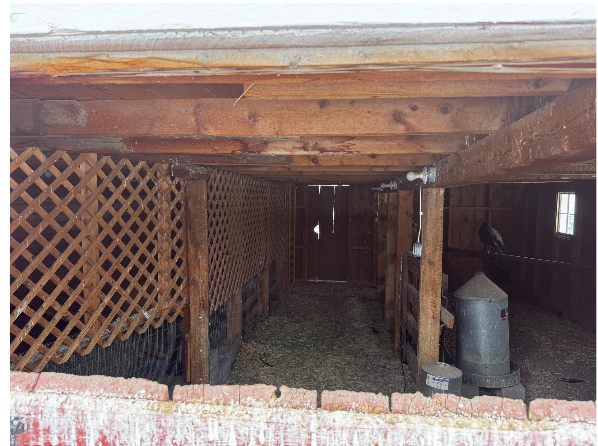
SOUTH BARN INTERIOR
