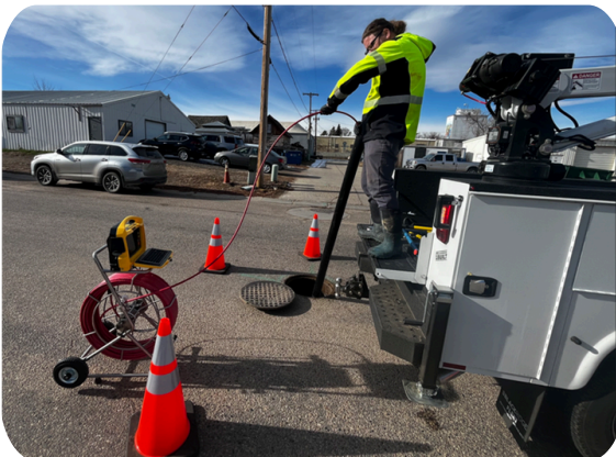
Crews used a push camera to inspect sewer lines on North 2 nd Ave. and confirmed the location and condition of manholes.
