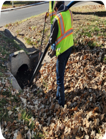
Streets crew jetting a culvert pipe under Welch Ave.
