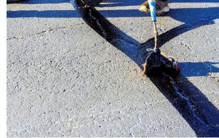
Crack Seal
