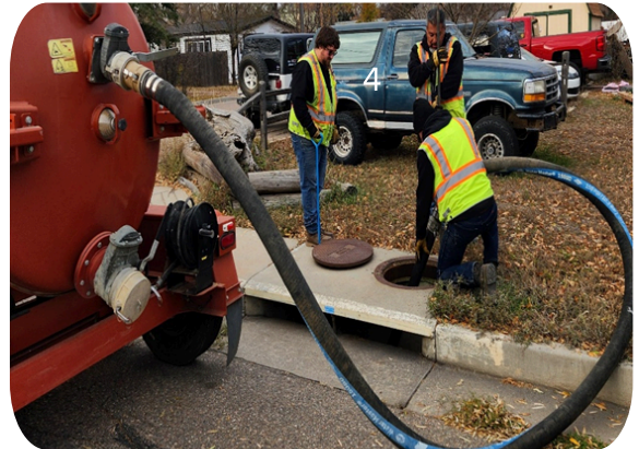
Cleaning out sediment from the storm drain basin on Franklin Ave.
