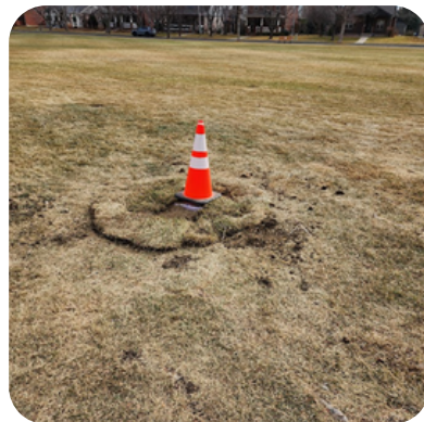
Crews releveled sod in areas that needed irrigation repairs.
