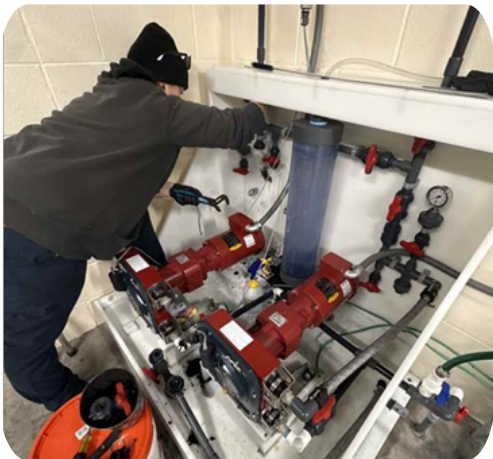
REC Operator performing the PAC Pump repair.
