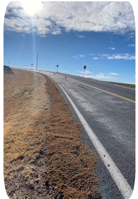
Road base was added to the inside edge of the roadway on County Road 11/42 to help motorists who might drive off the edge to reduce the risk of losing control of their vehicle.
