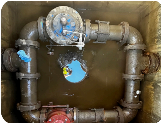
Water staff cleaned a Pressure-Reducing Valve (PRV). This piece of infrastructure reduces high water pressure to a safe level.
