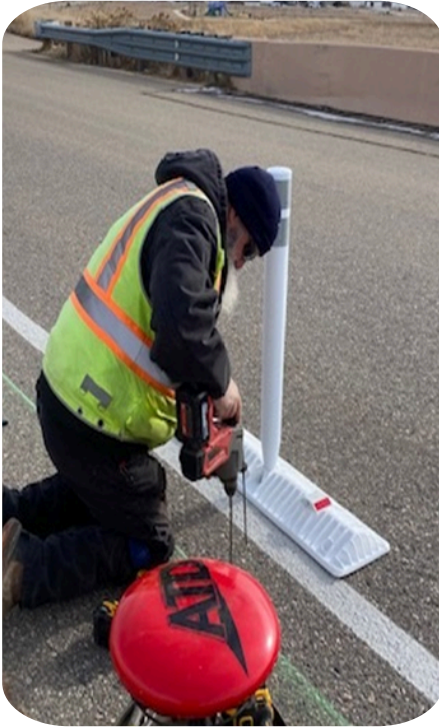
Streets crew installing delineation along the bridge on County Road 10E for pedestrian safety.
