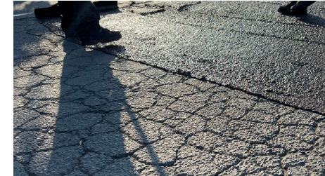
Slurry Seal
