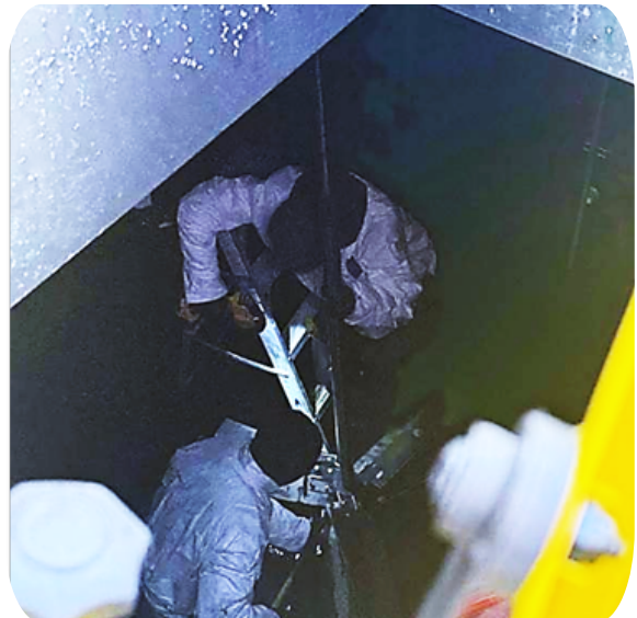
REC Operators performed the PAC Mixer repair.
