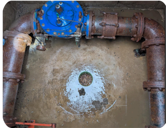
Water staff cleaned a Pressure-Reducing Valve (PRV). This piece of infrastructure reduces high water pressure to a safe level.
