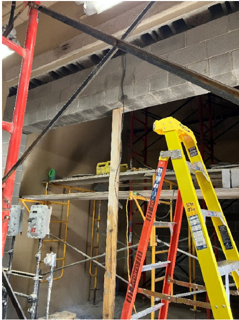
New Header in Headworks Building
