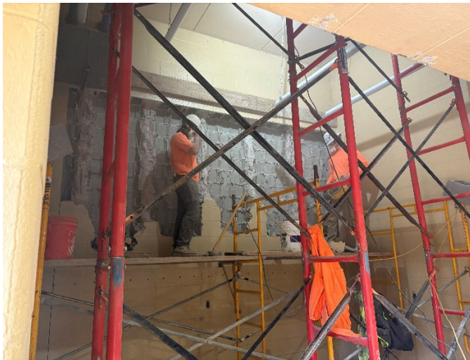
Headworks Building Block Removal
