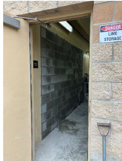
New Headworks Wall
