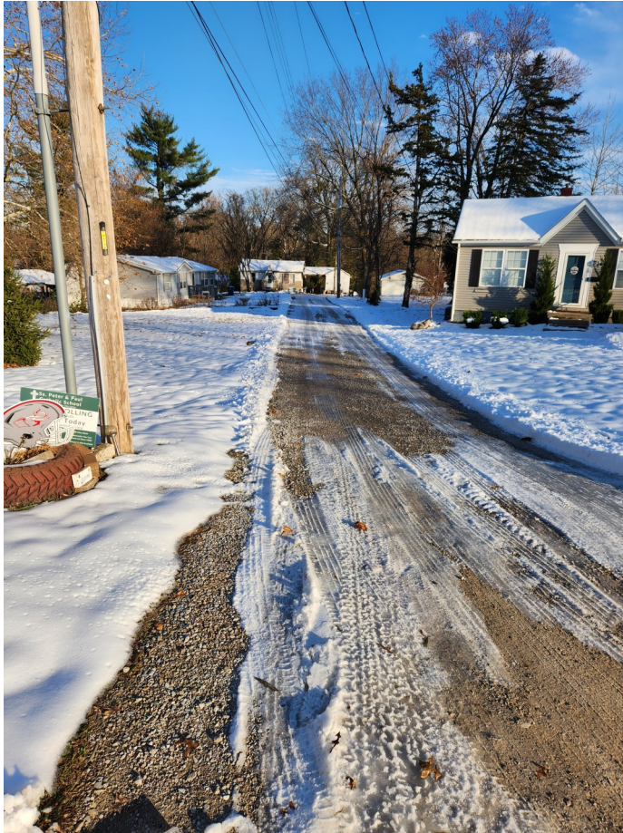
Photo of private drive entry off Ostle Drive
