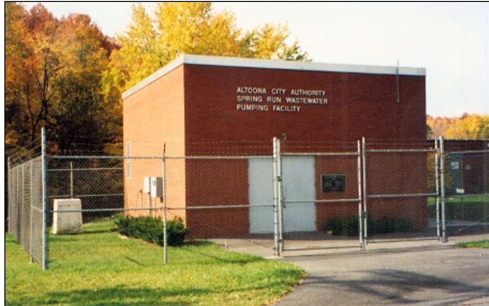
Spring Run Wastewater Pumping Station
