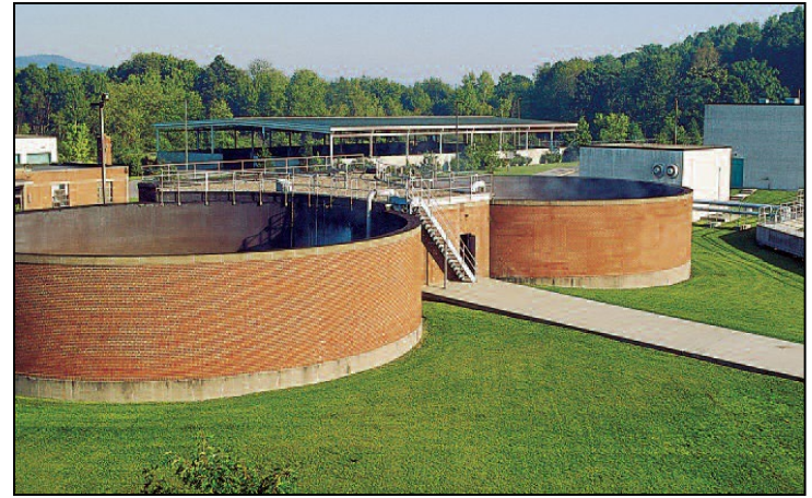
Sludge Digestion Tanks
