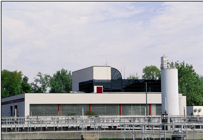
Operation & Control Building
