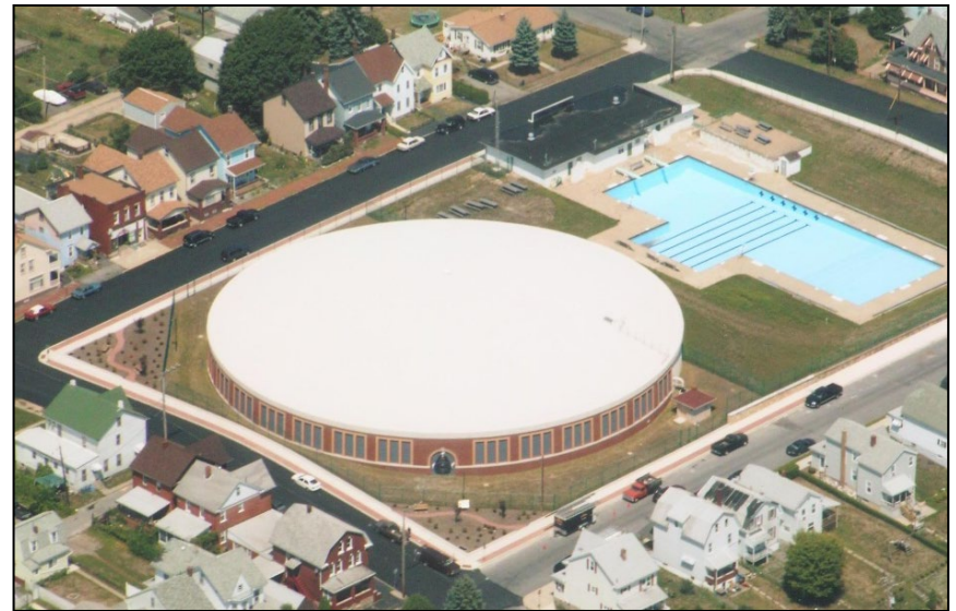
Prospect Water Storage Tank
