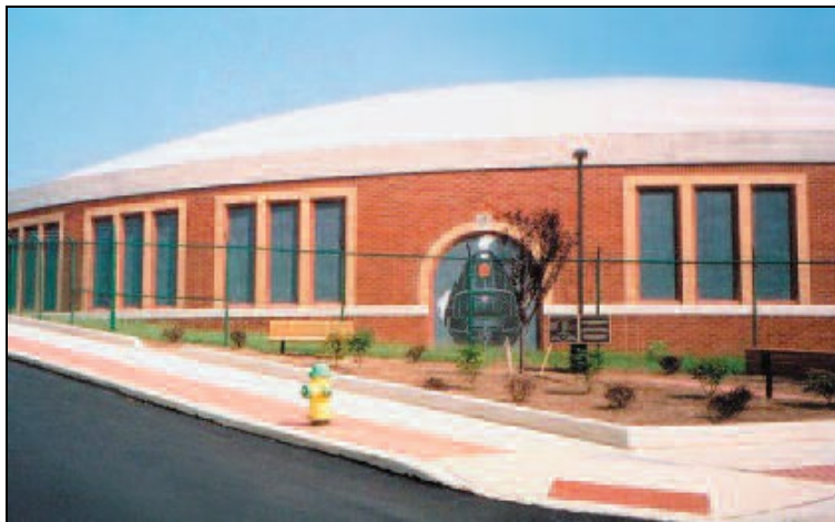
Prospect Water Storage Tank
