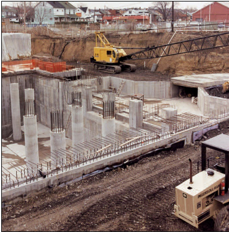
Storage Tank Construction, Bellwood Ave CSO
