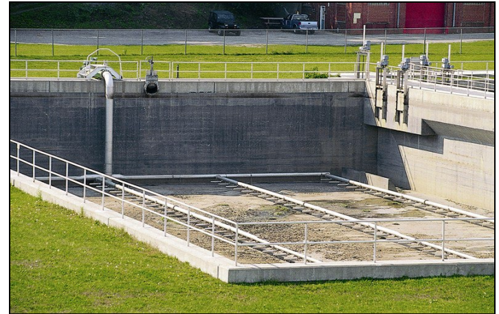
Overflow Storage Tanks
