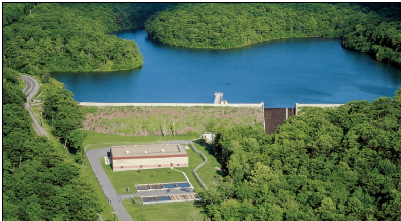
Kettle Reservoir & Water Treatment Plant
