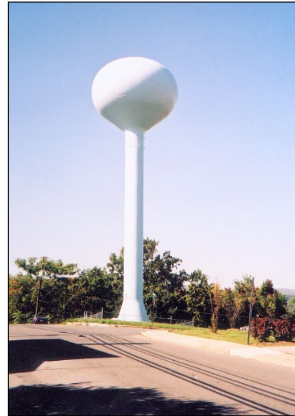
Fairview Hills Water Storage Tank
