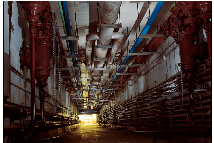
Pipe Gallery Tunnel
