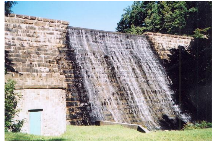
Blair Gap Dam
