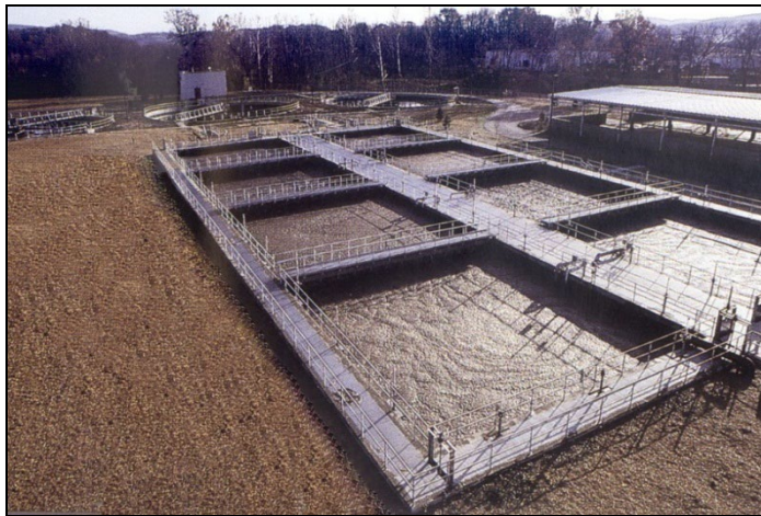
Ultraviolet Disinfection Tanks
