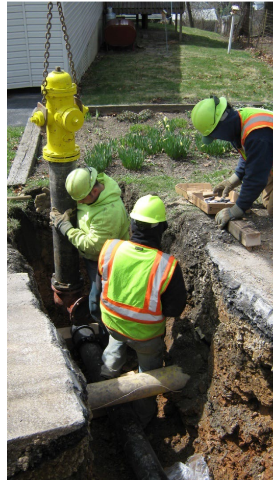
Installation of a fire hydrant
