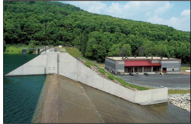
Plane 9 Dam & Water Treatment Plant
