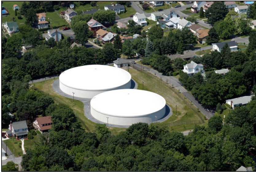
Oakton Water Storage Tanks
