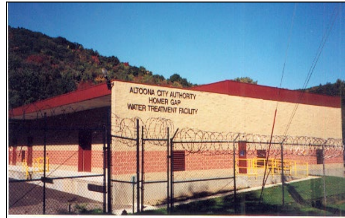
Homer Gap Water Treatment Plant
