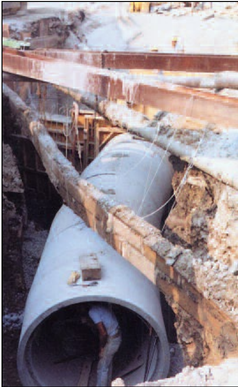
66" Combined Sewer Installation, Union Ave
