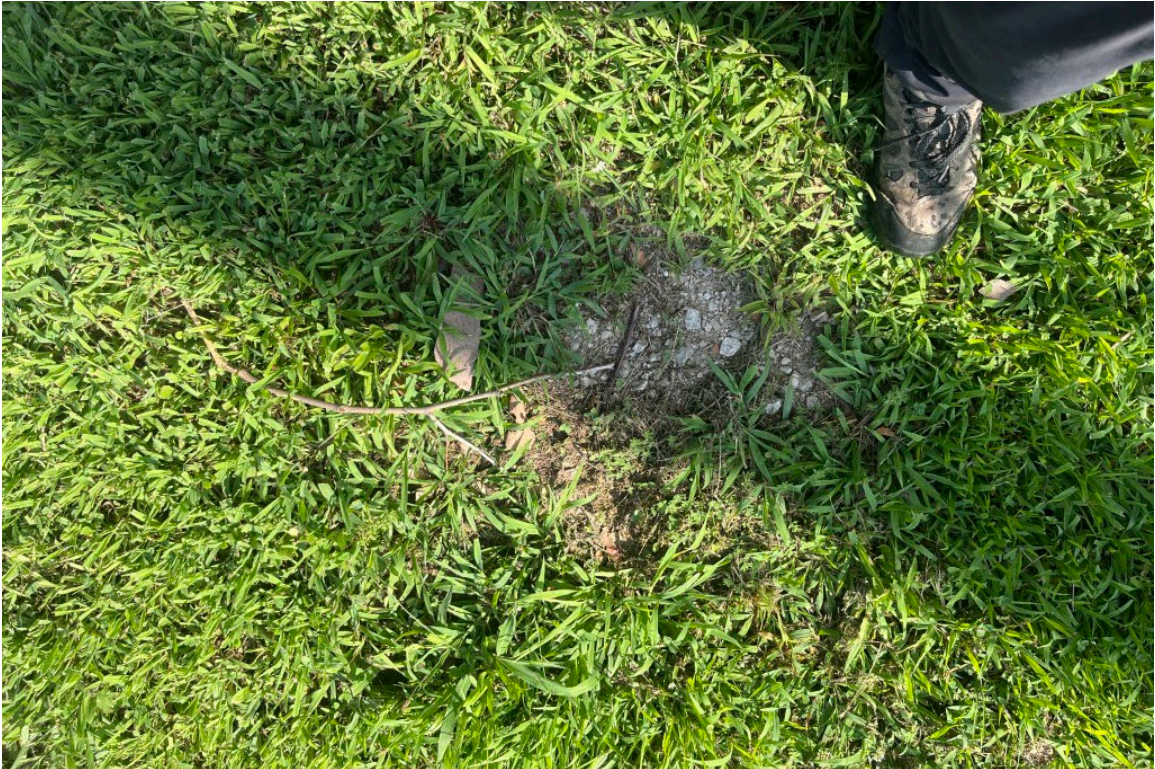
Photo 9. View of gravel around power substation.
