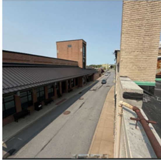
Roof Top- Street View
