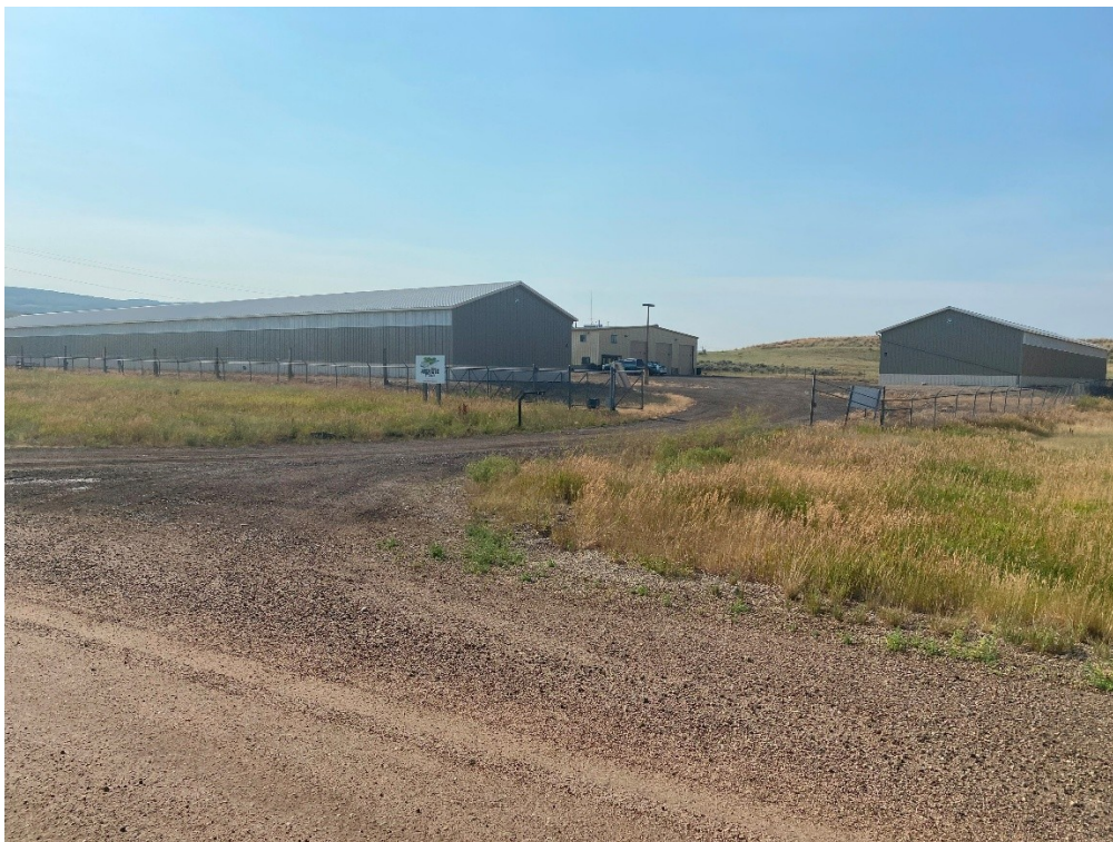
2. Entrance off of CR51B of Area 51B Storage
