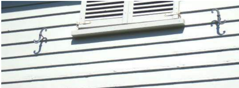
Wood siding is a lightweight skin for wood-framed buildings.
