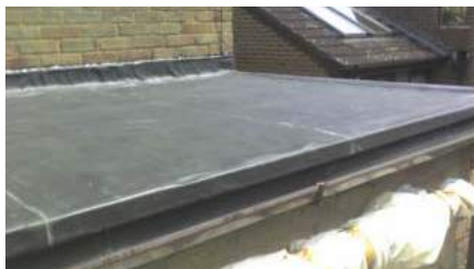
Rubber membrane roofing is limited to low pitches where not visible from the street.
