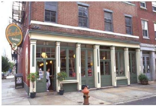
Traditional storefronts enter directly off the sidewalk.
