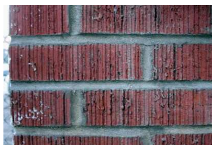
Wire-cut brick is a more recent innovation and the texture is not found in traditional construction.
