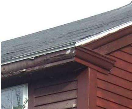
Gable end return on a tight rake condition.
