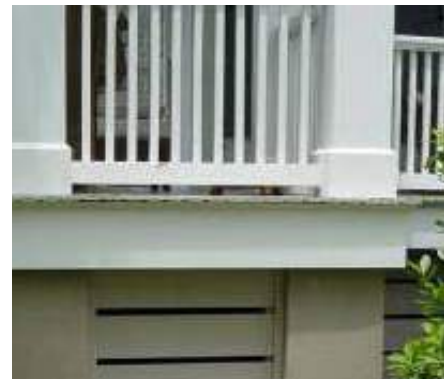
Avoid locating the column so that the base is flush with the decking. The column in this arrangement appears to cantilever from the structural pier and it appears that the column may fall off the deck. Also avoid placing columns without or misaligned to a structural pier.
