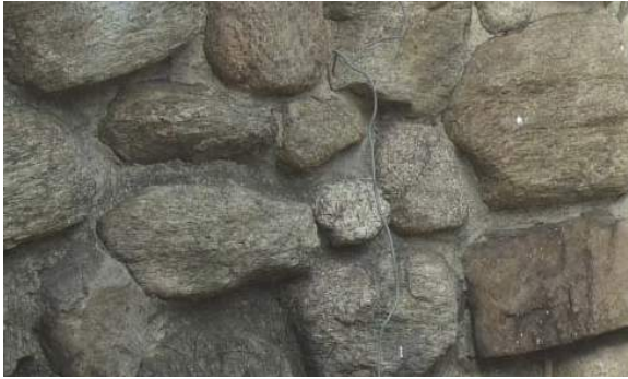
Masonry walls express strength and permanence.
