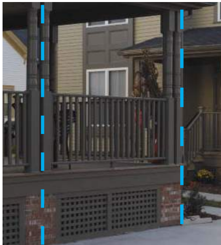
Align end columns to the corner of the pier and align intermediate columns to the center of the front face of the pier below.
