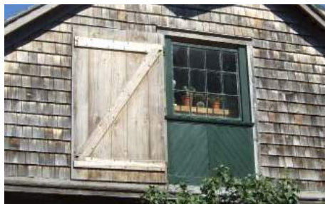
A barn shutter is sized so that a single leaf would cover the opening.
