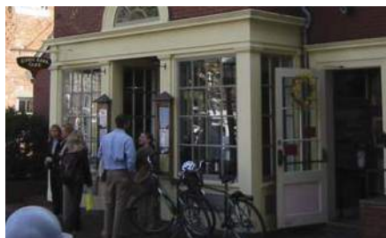
Vertical window proportions allow a traditional structural system with short spans and vertical piers to carry imposed loads to the ground.
