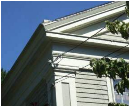
A continuous cornice at the gable end eliminates the gable return condition.
