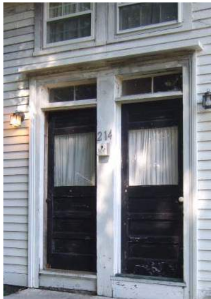
Casings are generally wider and more elaborate at the front entry to emphasize the door as a focal point.
