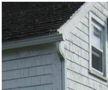
Gable end with minimal eave and rake detailing.
