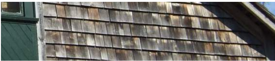
Traditional cedar shingles are arranged in horizontal courses with the bottom edges aligned. Shingles may be painted or left to weather naturally.
