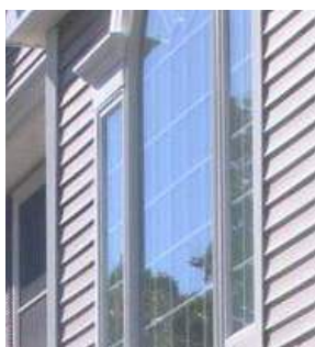
Windows with removable muntins or muntins embedded within the double glazing lack the depth that true muntins create. These “grids” are merely decorative and do not give the appearance of a muntin’s purpose.
