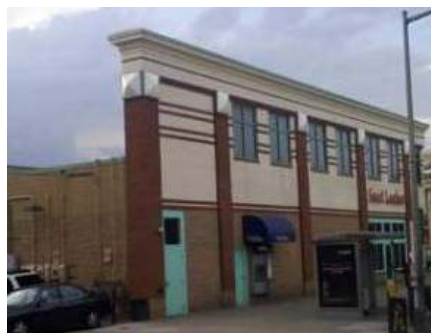
Parapet does not return on side elevation, appearing visually unstable.
