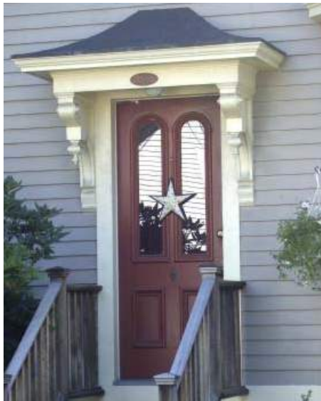
The entry door is clear and welcoming.
