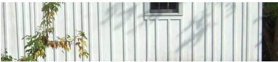
Traditional board and batten employs wide boards of a single or varied widths laid vertically with narrow batten strips to cover the joints.
