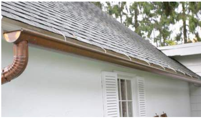
Quality materials, such as copper, can make gutters, downspouts and flashing into a decorative feature.
