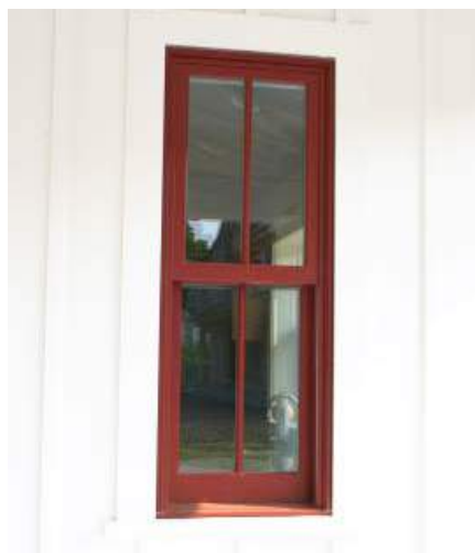
Windows may achieve higher energy efficiency by using simulated divided lite (SDL) technology. This gives the effect of traditional divided lites while allowing an air-tight seal between double panes of glass.
