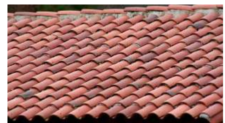
Avoid clay tile and other roofing types not found in the area. Avoid red, green and other colors not typical on traditional buildings.
