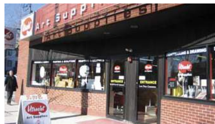
Horizontal window bands rely on hidden structural beams to span the long openings. These arrangements lack visual support for the stories above.
