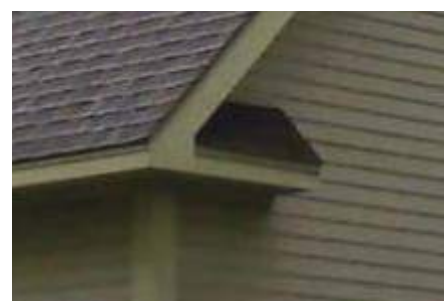
The pitch at the return significantly exceeds 1:12 – probably more like 12:12 in this case.
