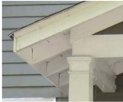
An eave with exposed rafter tails or sloping soffit needs no return.
