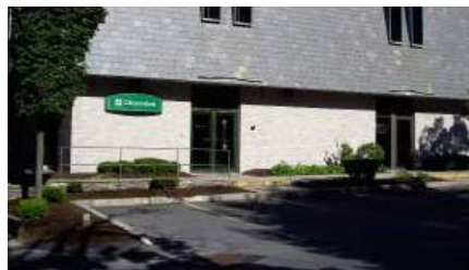
Residential foundation plantings force pedestrians away rather than inviting them to view wares.
