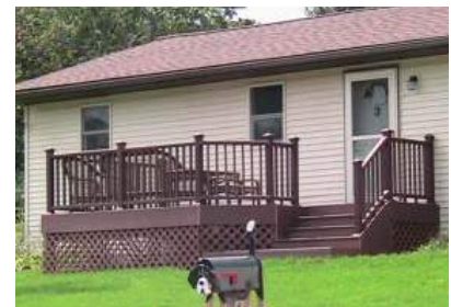
Open decks are not appropriate for the front of a home. Informal decks or patios may be constructed at the rear or side of a home.
