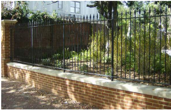
Fences and walls help identify distinguish public vs. private areas.
