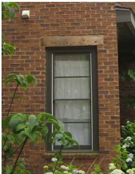
Traditional window casings are set into masonry openings.
