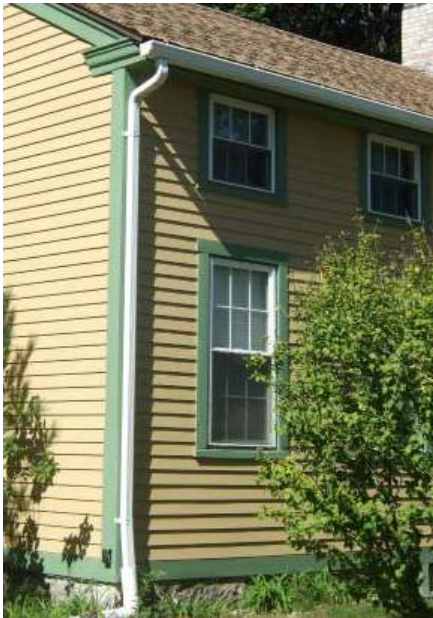
Trim is used at points of transition, such as between different materials at the foundation, roof and windows.
