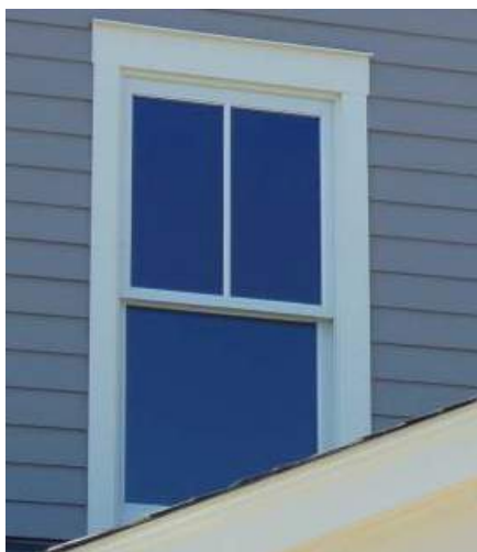
Windows may achieve higher energy efficiency by using simulated divided lite (SDL) technology. This gives the effect of traditional divided lites while allowing an air-tight seal between double panes of glass.
