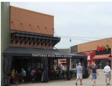
Unadorned parapets leave the facade feeling flat and unresolved.
