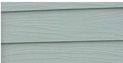
Faux wood grains on synthetic products add a texture that is not found in traditional wood clapboards.
