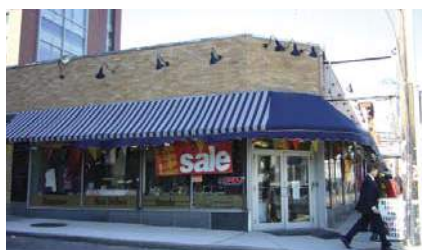
Horizontal window bands rely on hidden structural beams to span the long openings. These arrangements lack visual support for the stories above.
