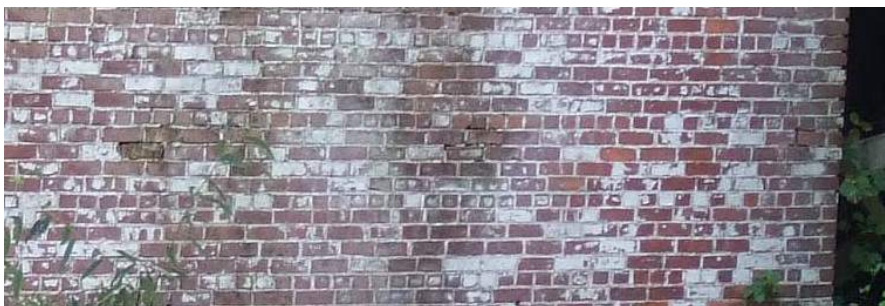
Brick is primarily found in foundations and mill buildings.
