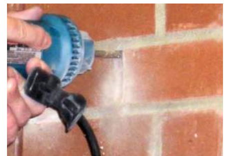
Avoid widening joints in the process of removing old mortar.
