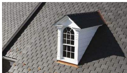
Avoid asphalt shingles designed to imitate shakes, slate or other materials. These products are poor representations of the traditional materials.
