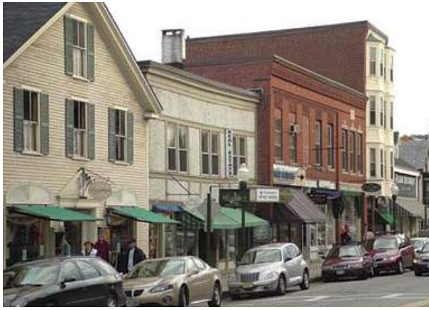
Flat roofs with parapets are common on main streets.
