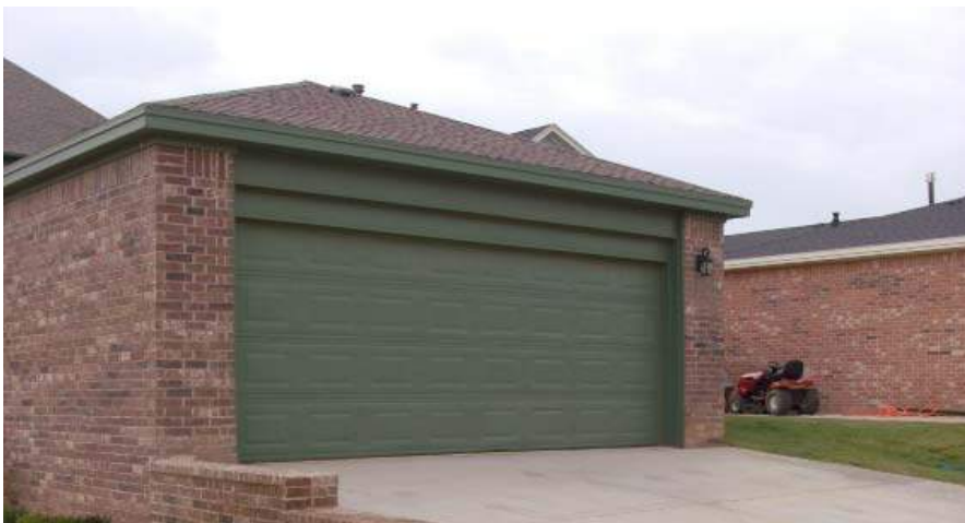
Avoid double-wide garage doors that do not have traditional proportions. These doors are oversized and out of scale with their surroundings.
