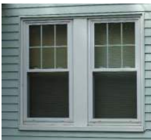
Openings without trim do not offer a transition between the siding and window.
