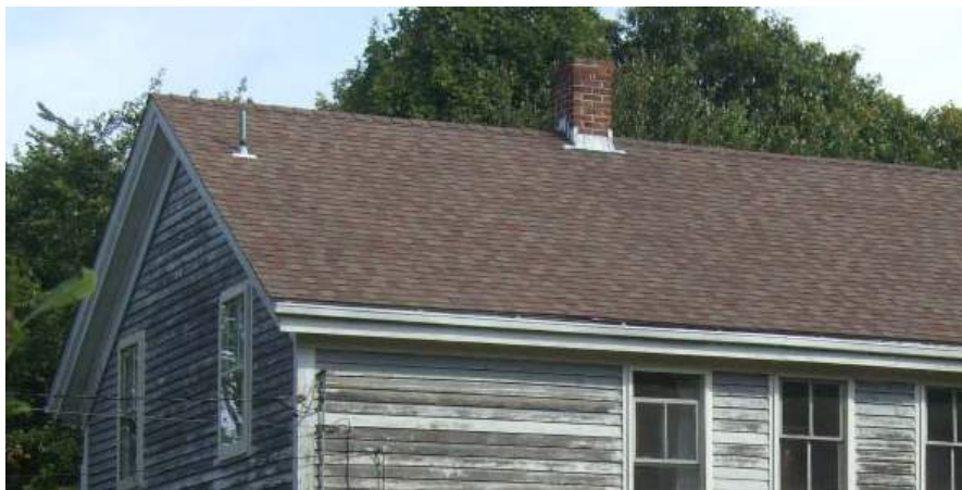
Most neighborhoods feature a range of roofing materials, including both 3-tab and architectural asphalt shingles in a range of colors.
