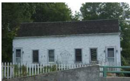
Split cedar shakes are appropriate roofing materials.
