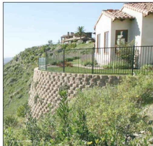
Figure 11: Typical Gravity Block Wall
